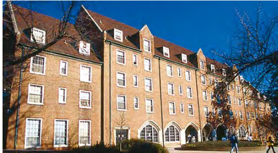
Strong Hall will be rebuilt to house EPS.
